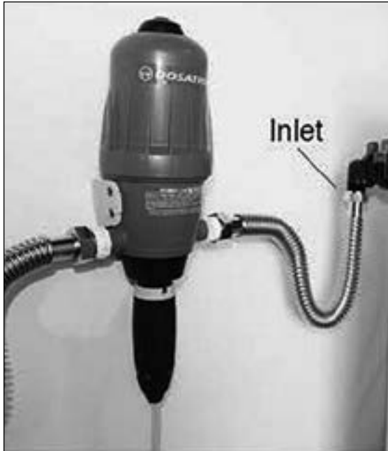
Dosatron Iron Tank Connection
